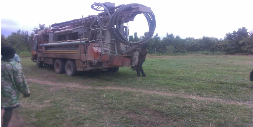
Fig.4- conveying of digging truck to the site
