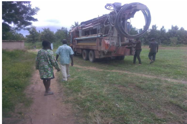
Fig. 26- Digging truck toiling through the bad road to the site
