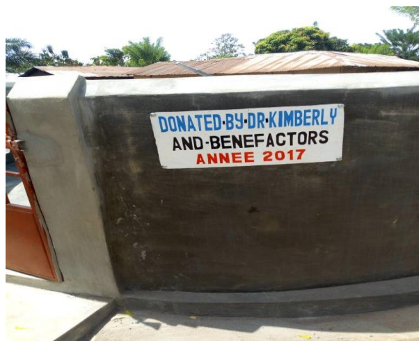
Fig. 27- Inscription plate fixed on the well's wall.
