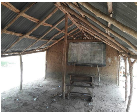
Fig. 2- Inside view of a classroom at the site
