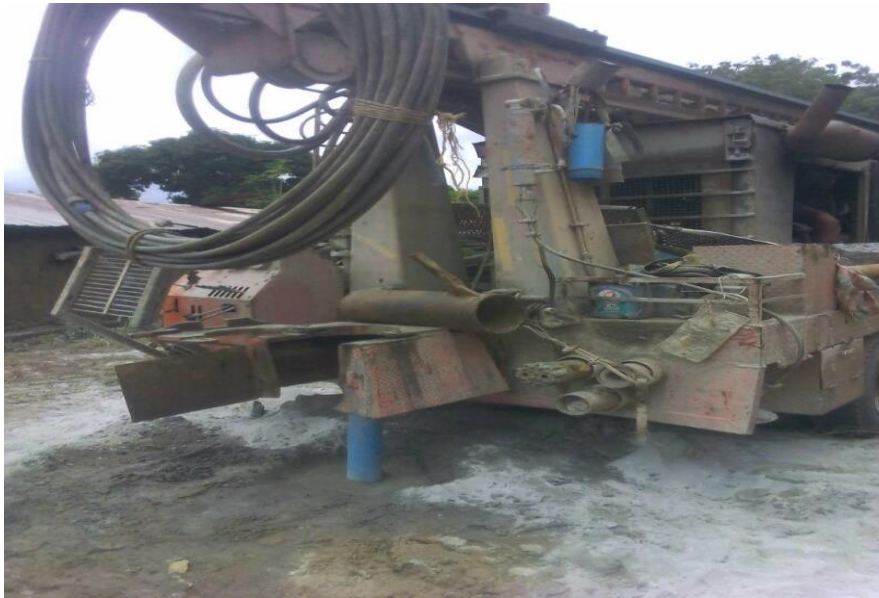
Fig. 5- Machine digging well
