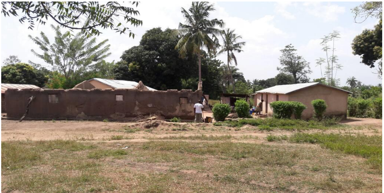
Fig. 1- View of site before digging of well.
