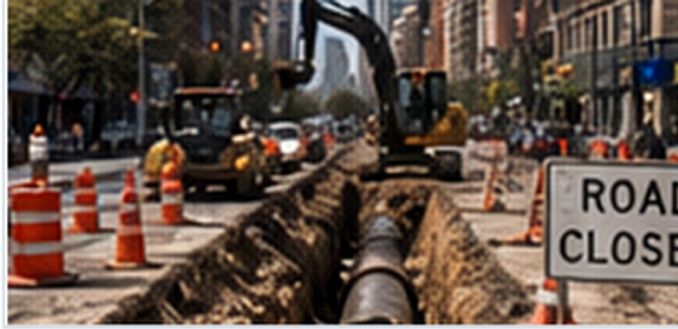
Figure 12.1. Street-level repair work shows how hidden infrastructure taxes reach city budgets, businesses, and residents.
