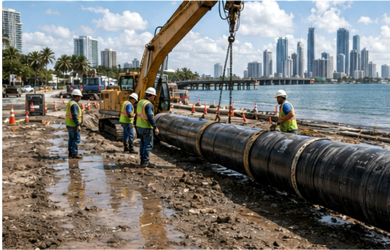
Figure 6.1. Coastal environments make material choice strategic by exposing corrosion, handling burden, and lifecycle cost in plain sight.
