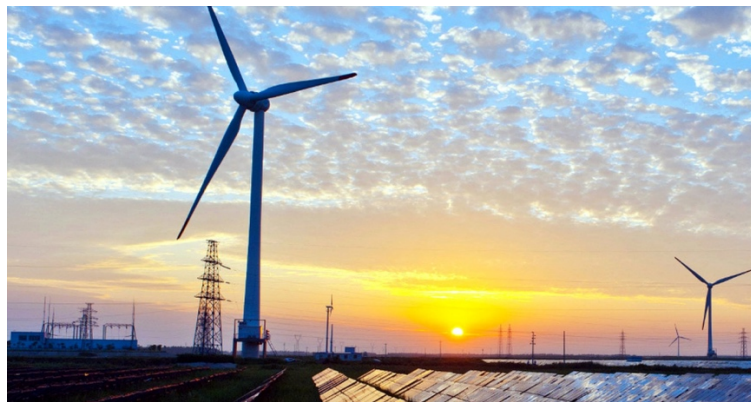
Figure 4.1. Renewable generation is essential, but clean power still depends on grids, storage, materials, water systems, and delivery infrastructure.
