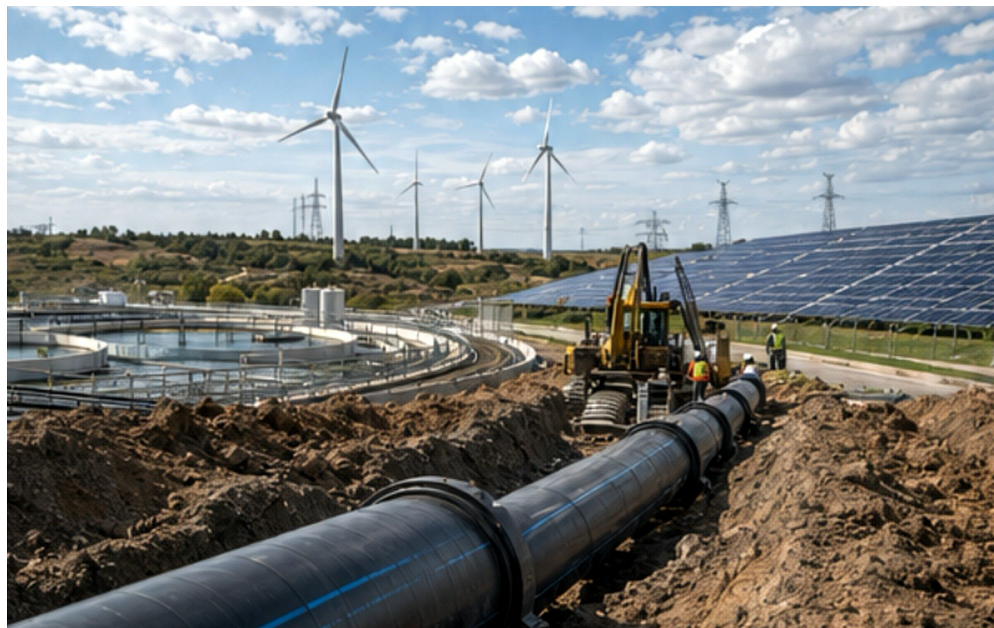
Figure 8.1. Bridge materials matter when they reduce leakage and lifecycle burden inside the systems society already depends on.
