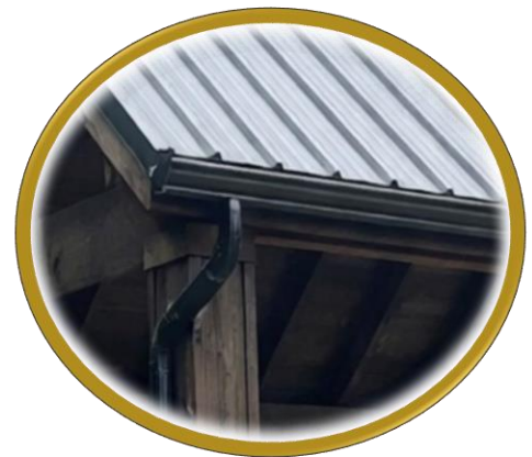
Black Metal Roof & Gutters
