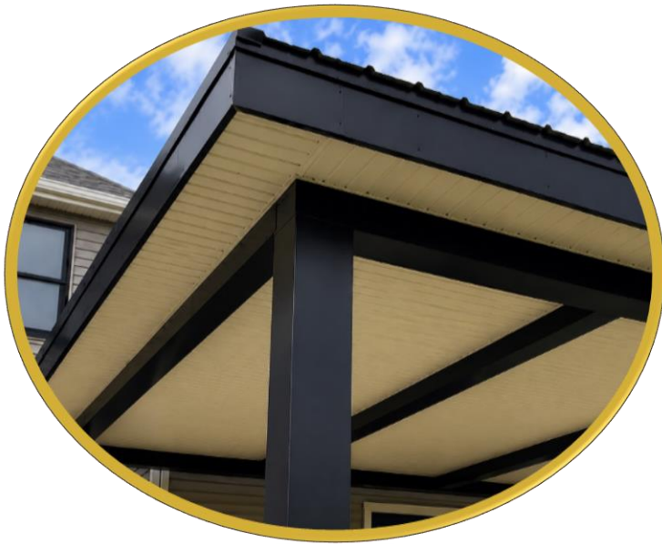
Finished Fascia & Soffit
