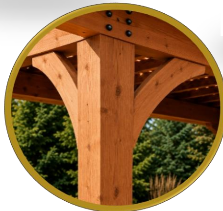
Arched Angle Bracing
