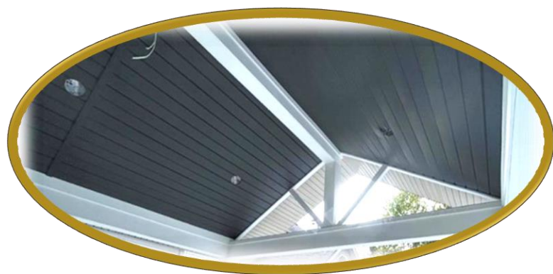
Finished Metal Ceiling
