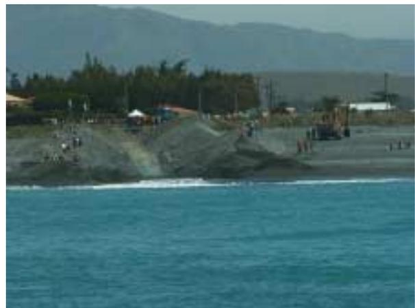
**Figure 5: Landing trench preparation at Kaikoura**
