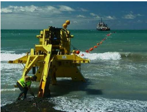
Clearly, trends toward deepwater burial below 2000 meters have abated. However, the trend toward deeper burial into the seabed has not. Burial increased from 0.6m in the early 1980's to 1.5m – 3m more recently. Even deeper burial is sometimes required in very soft soils, and
