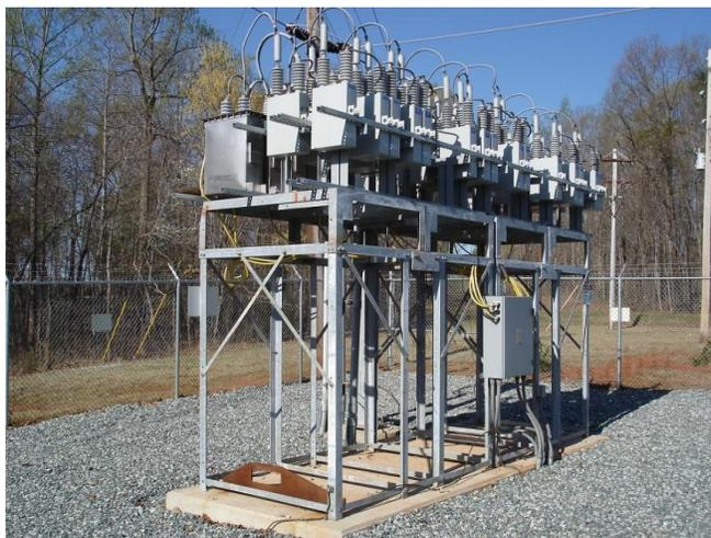
Figure 5 PEC SVC in Substation
